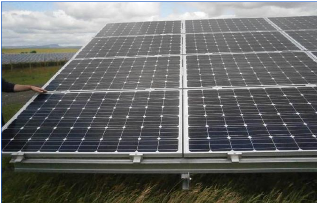
Figure 7-1 Typical Solar Panel Arrangement (showing expansion gaps)
